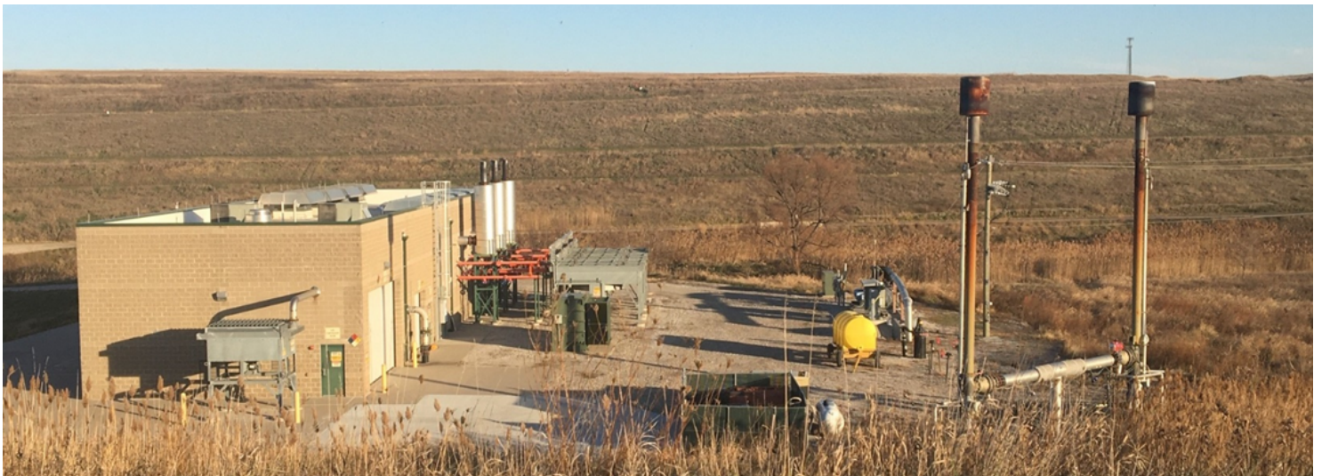
This photo shows one of two Methane Recovery Facilities at Metro Park East landfill.
