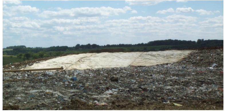
This photo shows daily cover using a tarp.
