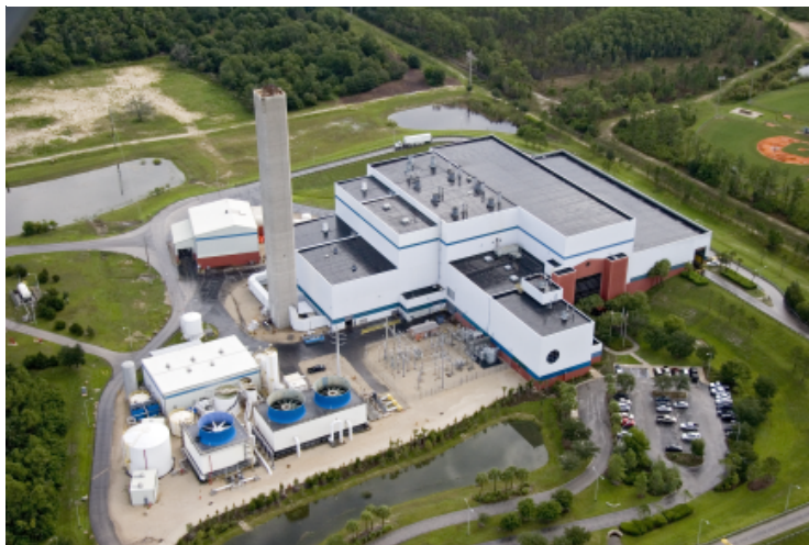
Figure 7. Mass Burn Facility, Florida
