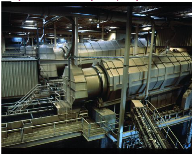
Figure 4. RDF Processing Facility, Virginia
